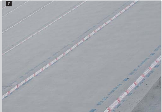
2 Ampatex® SB 130, formwork membrane, overlap taped with Ampacoll® XT.
