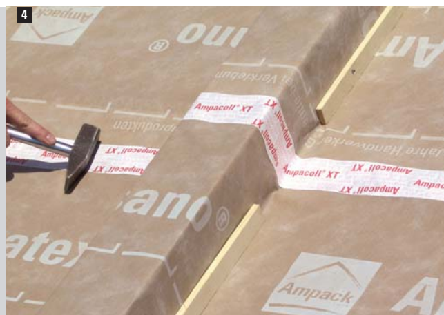
4 Moisture-variable Ampatex® Resano® vapour barrier, overlap taping with Ampacoll® XT.
