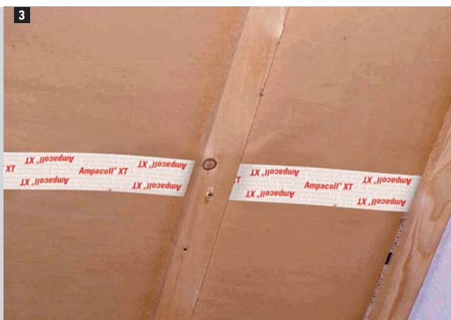
3 Sisalex™ 500, overlap taping with Ampacoll® XT.
