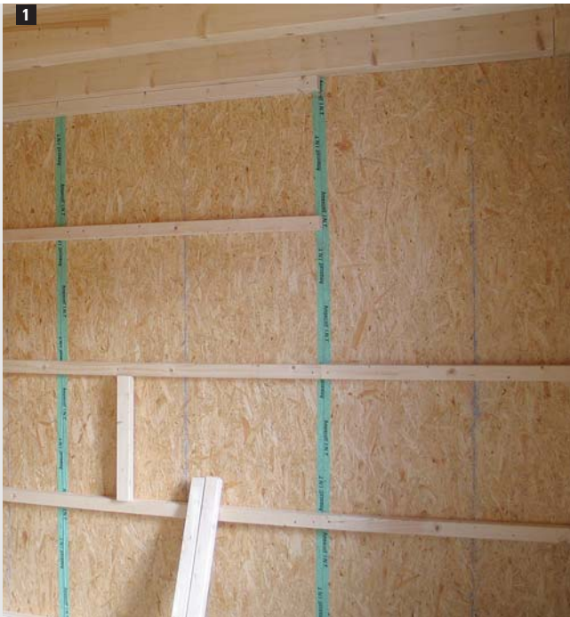
1 Airtight taping of DSB panels using Ampacoll® INT.
