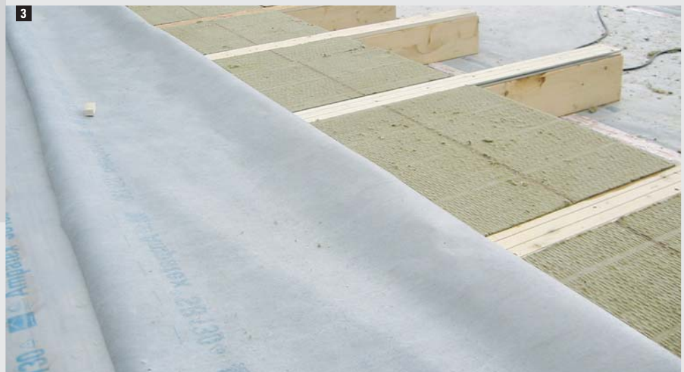
1-3 Rafter insulation using Ampatex® SB 130. Overlap taping using Ampacoll® XT.
