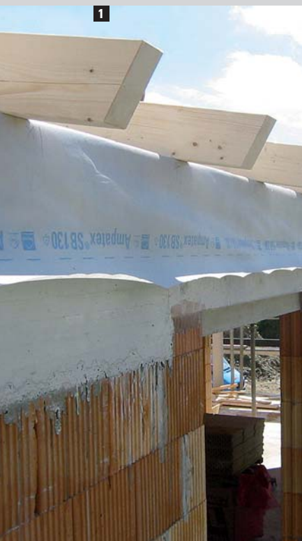
1-3 Rafter insulation using Ampatex® SB 130. Overlap taping using Ampacoll® XT.
