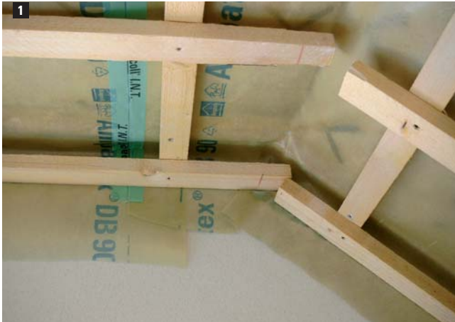
1 Ampatex® DB 90, overlap taped with Ampacoll® I.N.T.
